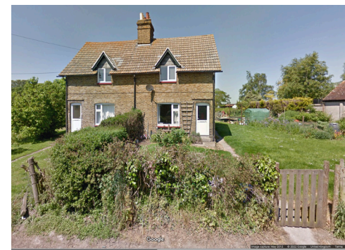
1. Semi-detached property with yellow, buff brick walls, clay tile roof and pitched dormers.
