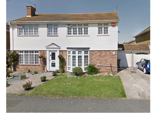
4. 2 storeys, detached property comprised of ground floor light red brick walls and first-floor weatherboard cladding, vertical bay window feature. The buildings are set back from the edge of the pavement by 6m and provide a side parking drive and integral garage.
