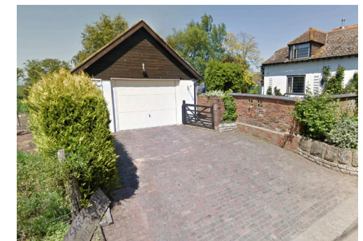
2. St Mary's Hoo - Gable-ended side garages with driveways.
