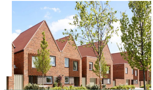
Horsted Park, gable ended frontages
