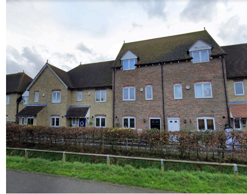
3. 2-2.5 storey red and yellow brick terrace with gable-ended/pitched roofs, pitched roof porches, and dormers. A white picket fence and hedges mark the plot boundary.
