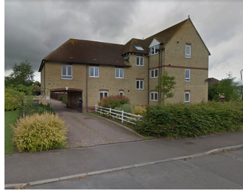
2. 2-2.5 storey yellow brick flats and terrace with a hip clay tile roof and varying roofline. The plot has a rear parking courtyard with garages for the residents of the flats and terrace. Hedges and a white picket fence demarcate the plot boundary.
